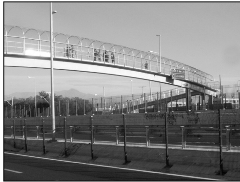
(c) Pedestrian overpass
