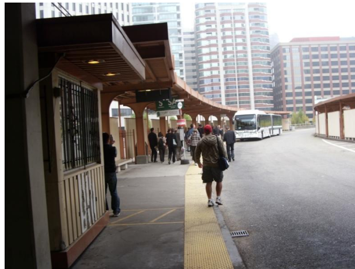
Figure 1 – Former Transbay Terminal in San Francisco – an unlikely launching pad for a 21 st century mass transit financing revolution...? (author 2008)
