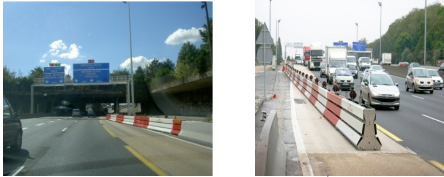
Fig. 2. The weaving A4-A86 section, eastbound with the 5 th lane, open and closed
