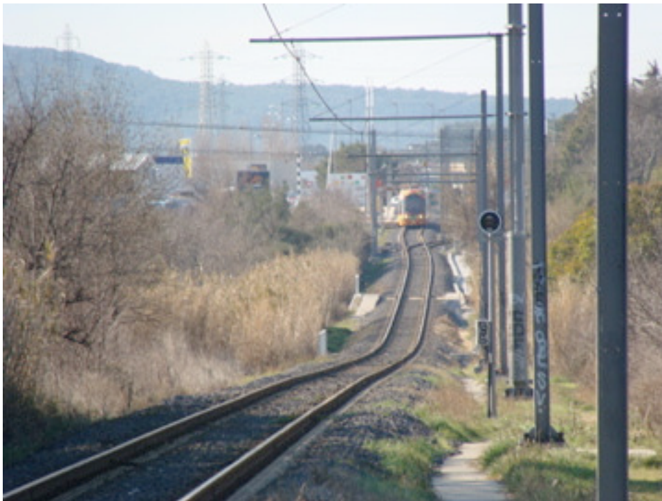
Picture 2 : View of line 2 of the Montpellier tramway on a former railway line section between Les Sabines and St-Jean de Védas (Author: Pierre Zembri)
