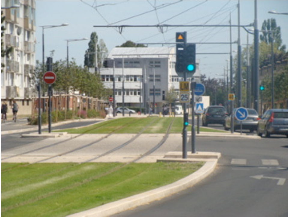
Picture 1: reduced speed across intersections : an illustration along the new line B in Orléans. Another signpost at the rear shows a higher speed limit for the next section of the line (40 kph) (author: P. Zembri)
