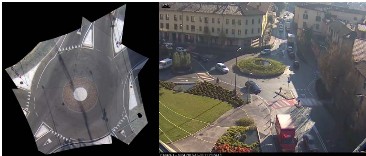
Figure 4 – Aerial view of the Chiari and Sarnico roundabouts
