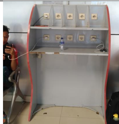
Figure 3. One of the facilities provided at station
