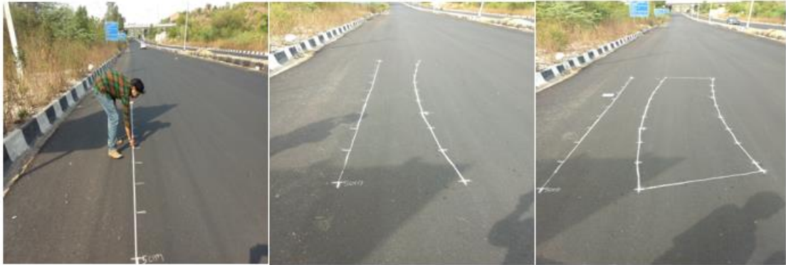
Fig 9. Plotting Contour of Curved Speed Hump
