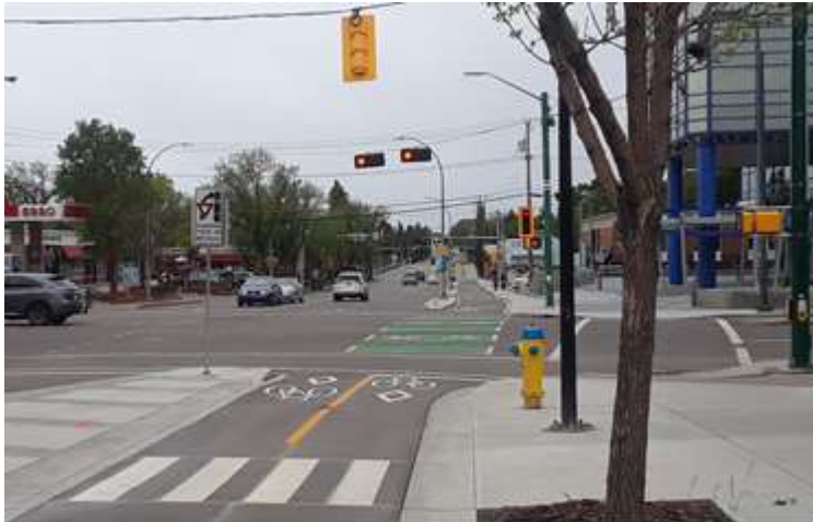
Fig. 6. Separate lanes for bicycles, pedestrians and automobiles
