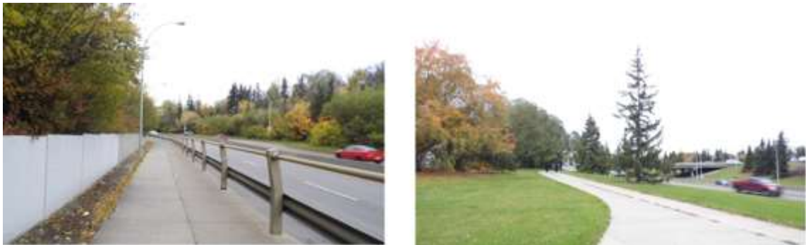
Fig. 10. Engineering controls (guardrail) as shield, and considerable buffer for vulnerable road users
