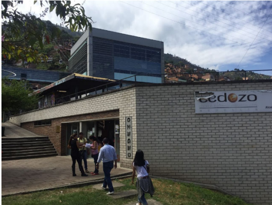
Fig. 12. CEDEZO near Santo Domingo station
