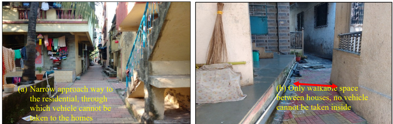
Fig. 2. Houses with very less approach width (Location - (a) AL/H type, Sector 6, Airoli, (b) Diwale Gaathan Area (Belapur CBD))
