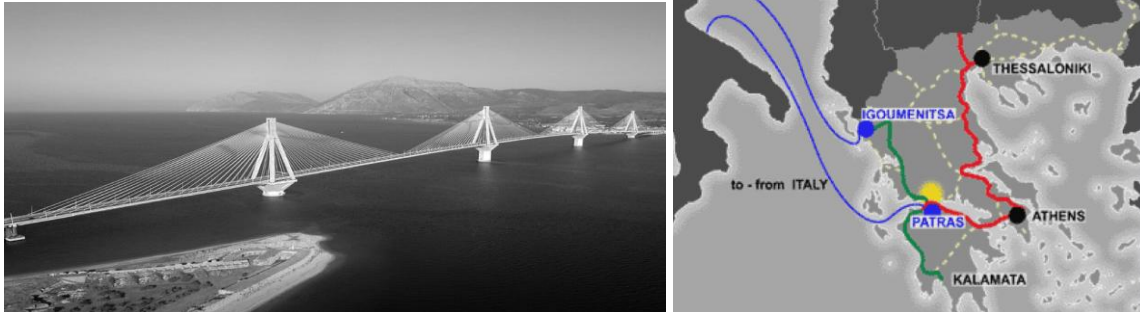
Figure 1 - The Rion – Antirion Bridge and the national road transport network its location (source: www.iabse.gr accessed on 16/07/2009 and Pilassi du Rausas, 2006)
