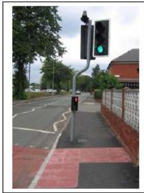
Figure 1 Puffin Type Control showing overhead detectors and nearside pedestrian signal
