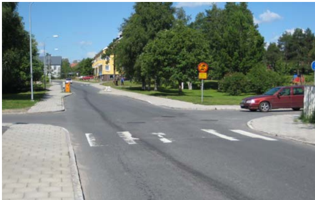
Figure 5. Backgatan, viewed towards north.
