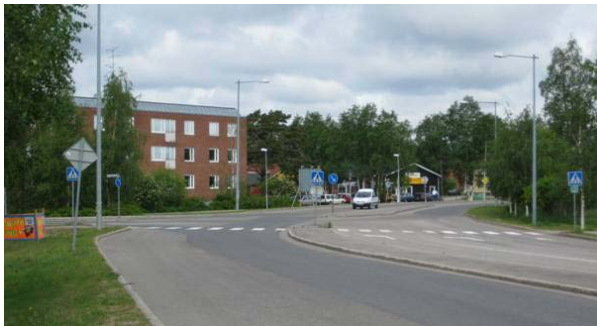
Figure 14. Centrumvägen at Postgatan, view towards west.
