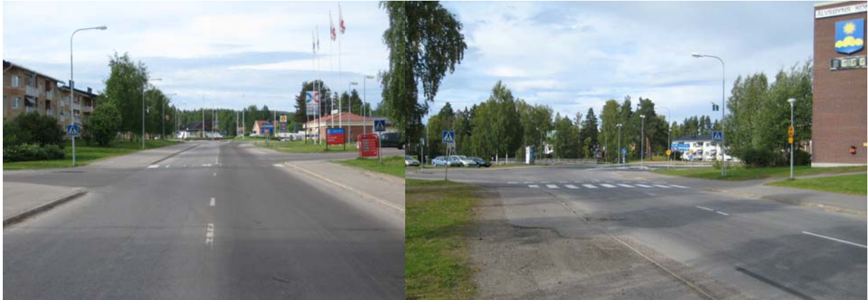
Figure 9. South pedestrian crossing to the left, view to the south. North pedestrian crossing to the right, view to the north.
