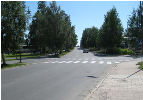
Figure 3. Skeppsbrogatan, viewed towards south.
