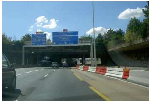
Photo 2. Moveable barrier on the hard shoulder running lane of A4-A86
