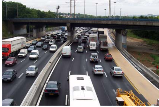
Photo 1. The hard shoulder running lane on the A4-A86 section
