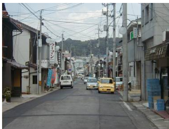
Figure 2 Conditions before Street Improvement Project
